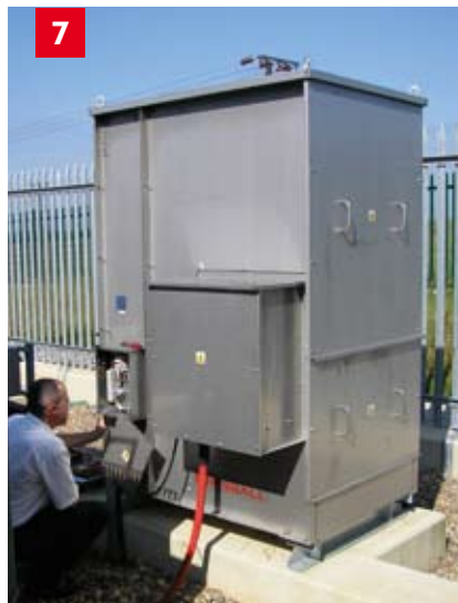
6 Resistor, on load isolator, surge arrestor & CT
