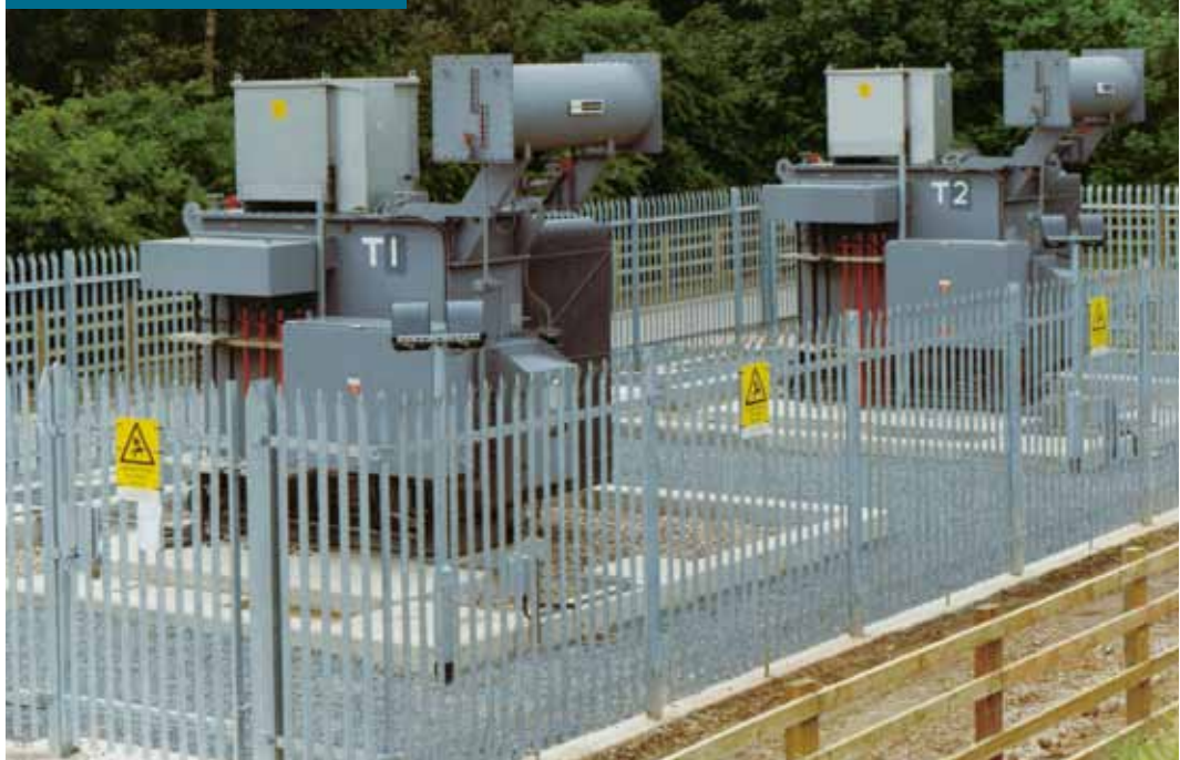
Transformer mounted NER rated 11kV, 1000A for 10 seconds.
